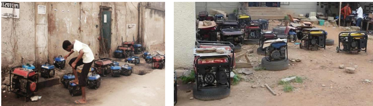
Pic 2: Erratic electricity in Nigeria and household reliance on generators Source: Pulse.ng, Punch Newspaper (2024)
